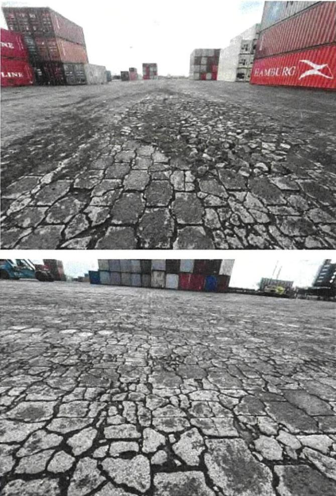
The image contains two photographs showing a paved area with cracked asphalt. The top photograph shows a perspective view of the cracked pavement leading towards stacks of shipping containers. The bottom photograph is a closer view of the cracked asphalt. The containers in the background are various colors, including red and blue, and some have logos like 'HAMBURG' and 'LINE'.
